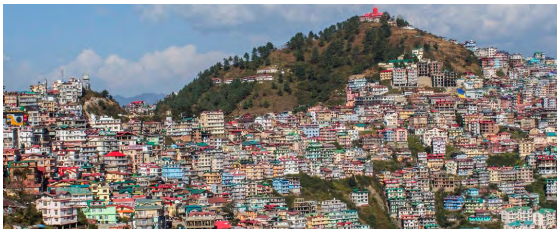
Sanjauli area of Shimla city dotted by recently done construction of RCC Buildings
